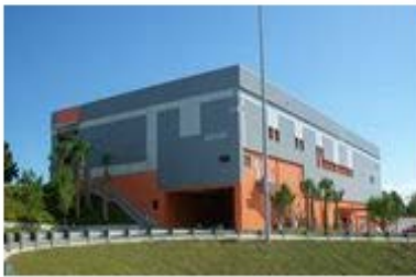
South County solid waste transfer Station in Delray Beach
